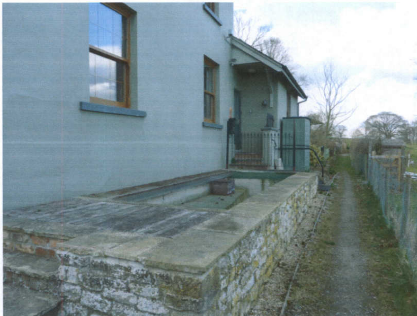
East elevation viewed from private footpath from Water Lane serving Station House and 1-6 Station Cottages
